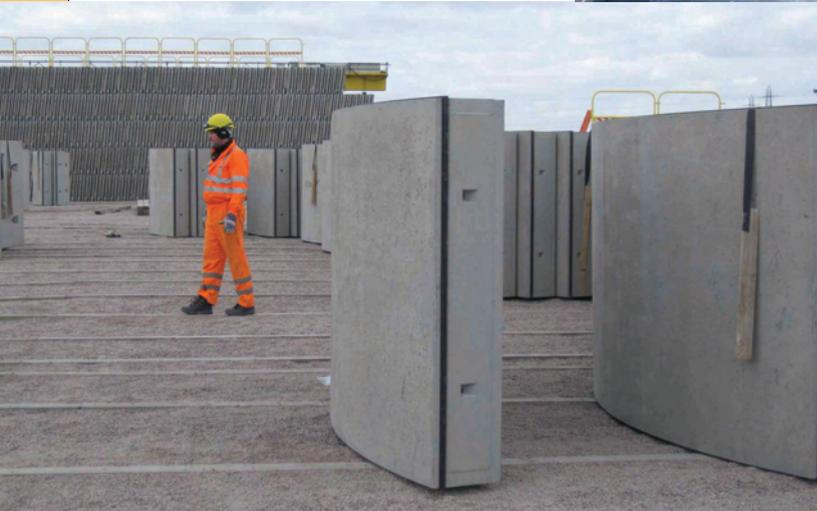
**Left: The yard at the Ridham Precast facility begins to fill up with stacks of rings for the Lee Tunnel**
