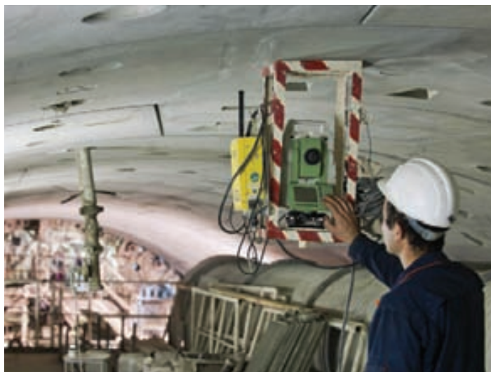
Above: 2010 - First microtunnelling curve drive in the US successfully completed with a radius of 414m and precisely guided by a VMT navigation system.
