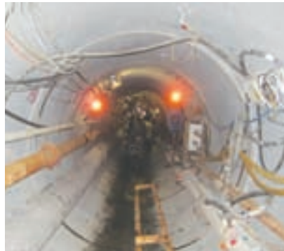
A view of the reference prisms used in Phase 2 of the project
