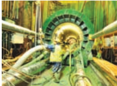
Looking into the tunnel from the starting shaft
