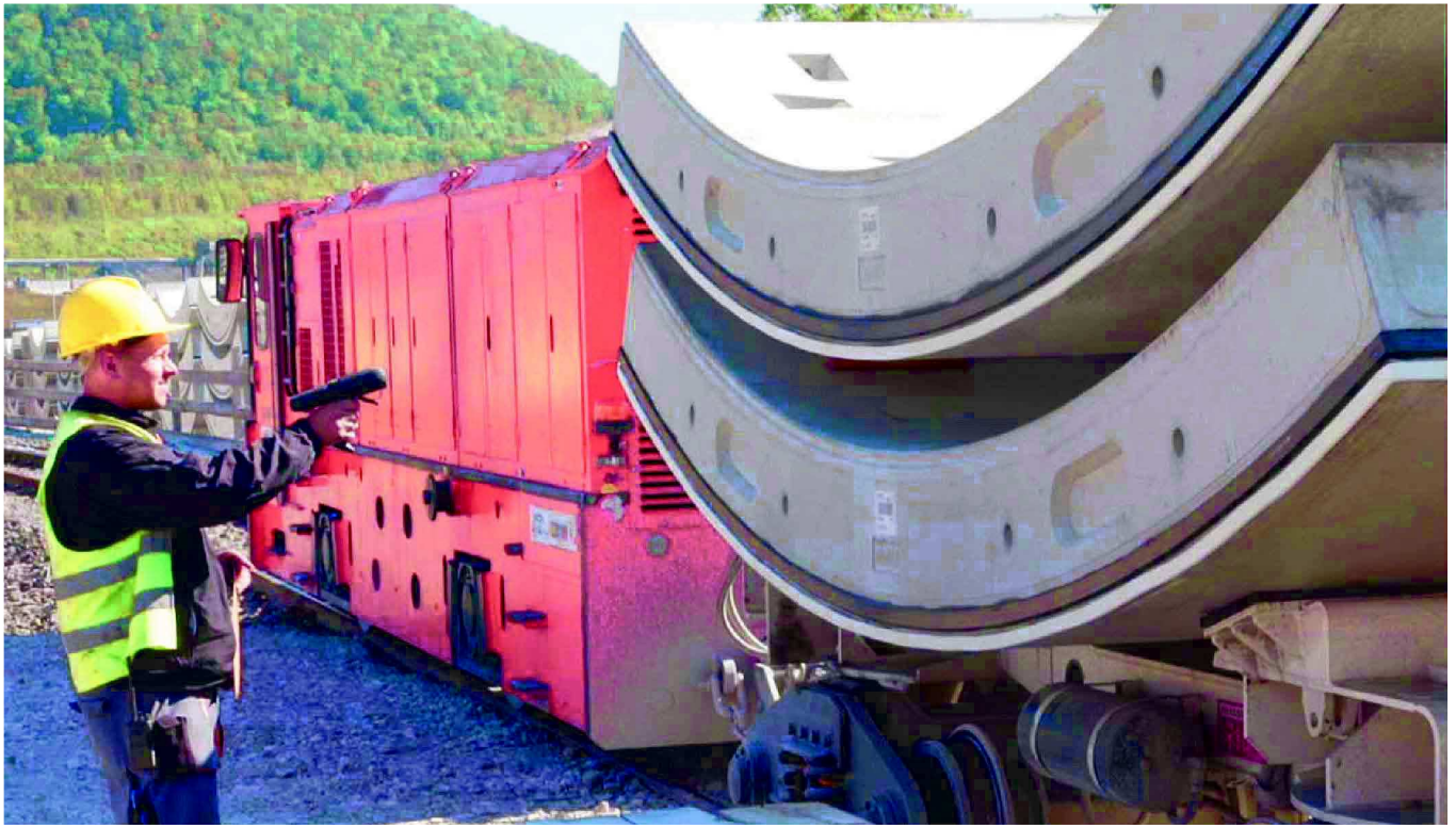
Information on segments is available via barcodes and RFID tags.
